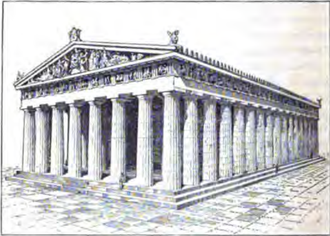
FIG. 185. RESTORATION OF THE PARTHENON, AS IT WAS IN THE FIFTH CENTURY B.C. (AFTER THIERSCH AND MICHAELIS)
