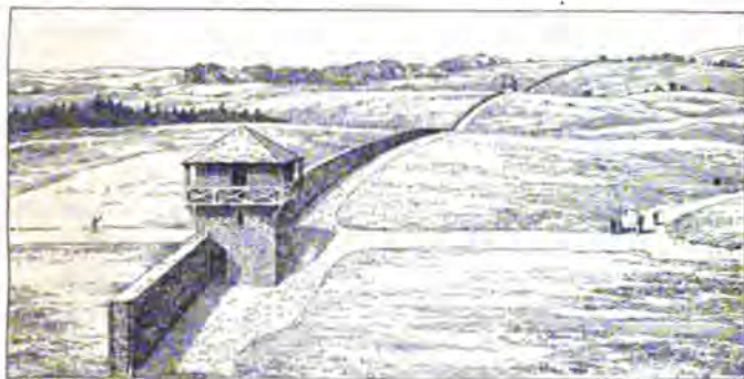
FIG. 252. RESTORATION OF THE ROMAN FORTIFIED WALL ON THE GERMAN FRONTIER
